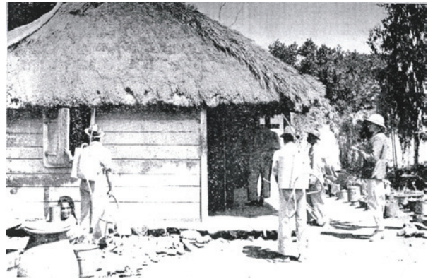
Figure 8. A team proceeding to spray a hut with residual insecticides
